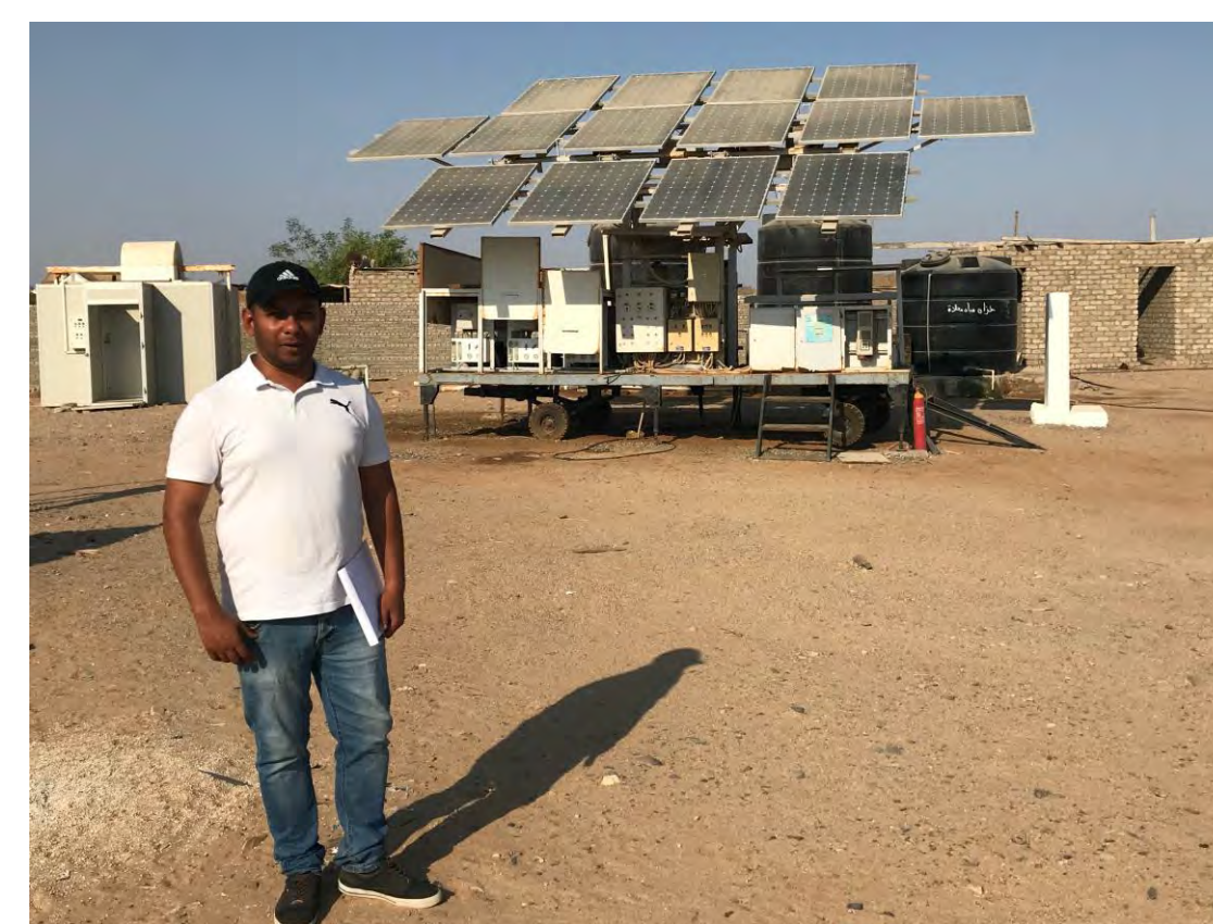
Figure 1: The imbedded reverse osmosis unit empowered by solar panels
